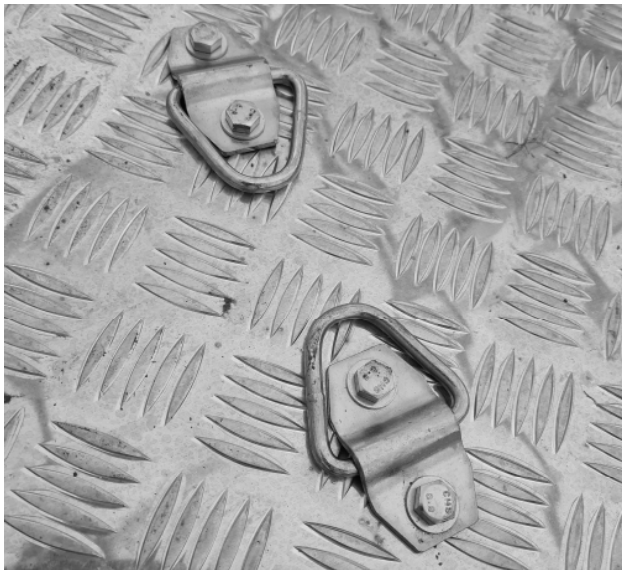
Figure 4.15 – Fall Restraint Points
